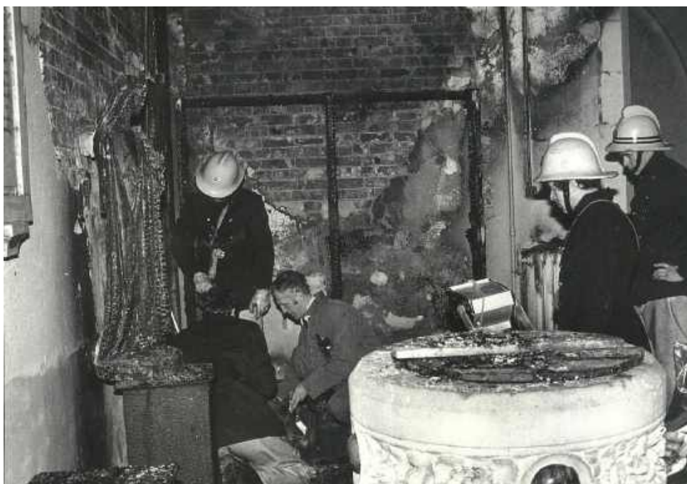
Picture on the left: Fire damage to St Pancras, Christmas day 1985
